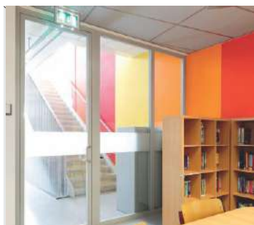
Fire Protective Doors
