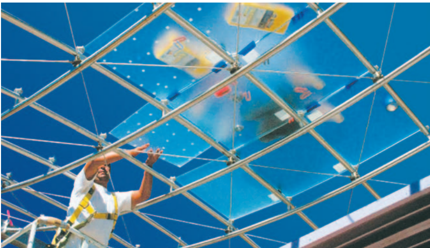
SentryGlas® Plus Installation: Overhead Glazing
