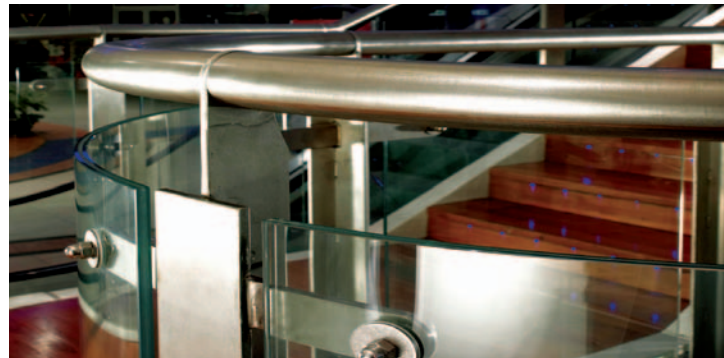
SentryGlas® Plus Installation: Stair Rail
