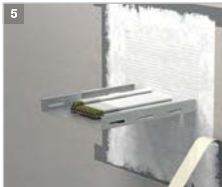
5 Coat the complete surface inside the mask with ROKU® MFC 100 to a total thickness of at least 1 mm.
