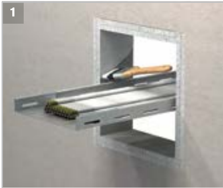
1 Clean aperture and remove all loose parts. Cover the surface of the aperture with ROKU® MFC 100 coating.
