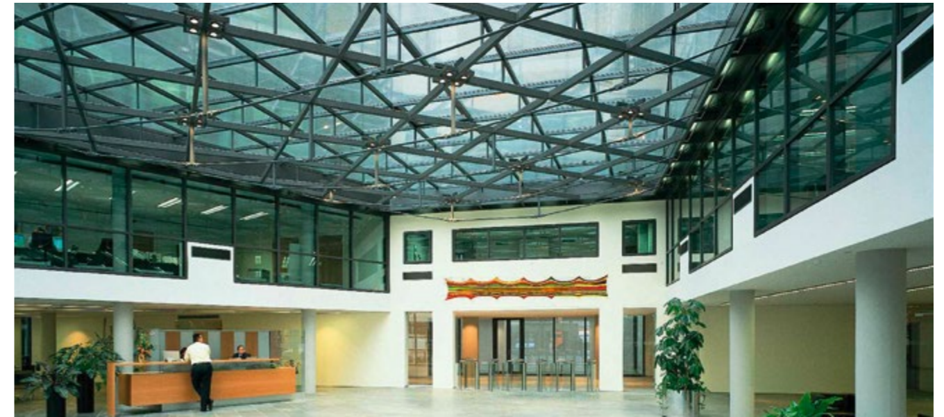
Westdeutsche Immobilienbank in Mainz, Fire-resistant roof G30 built by Krause Company PYRAN® S Special glass from SCHOTT.
